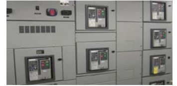
Retrofill before and after
