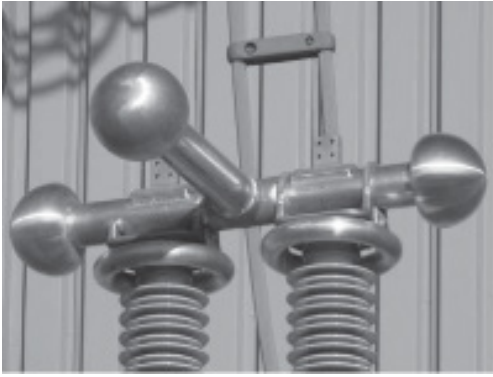
Figure 2.2-6 Welded T Connection and Bus Supports
