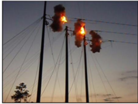
Figure 2.2-10 Multiple IMPLO® deadends being installed simultaneously.
